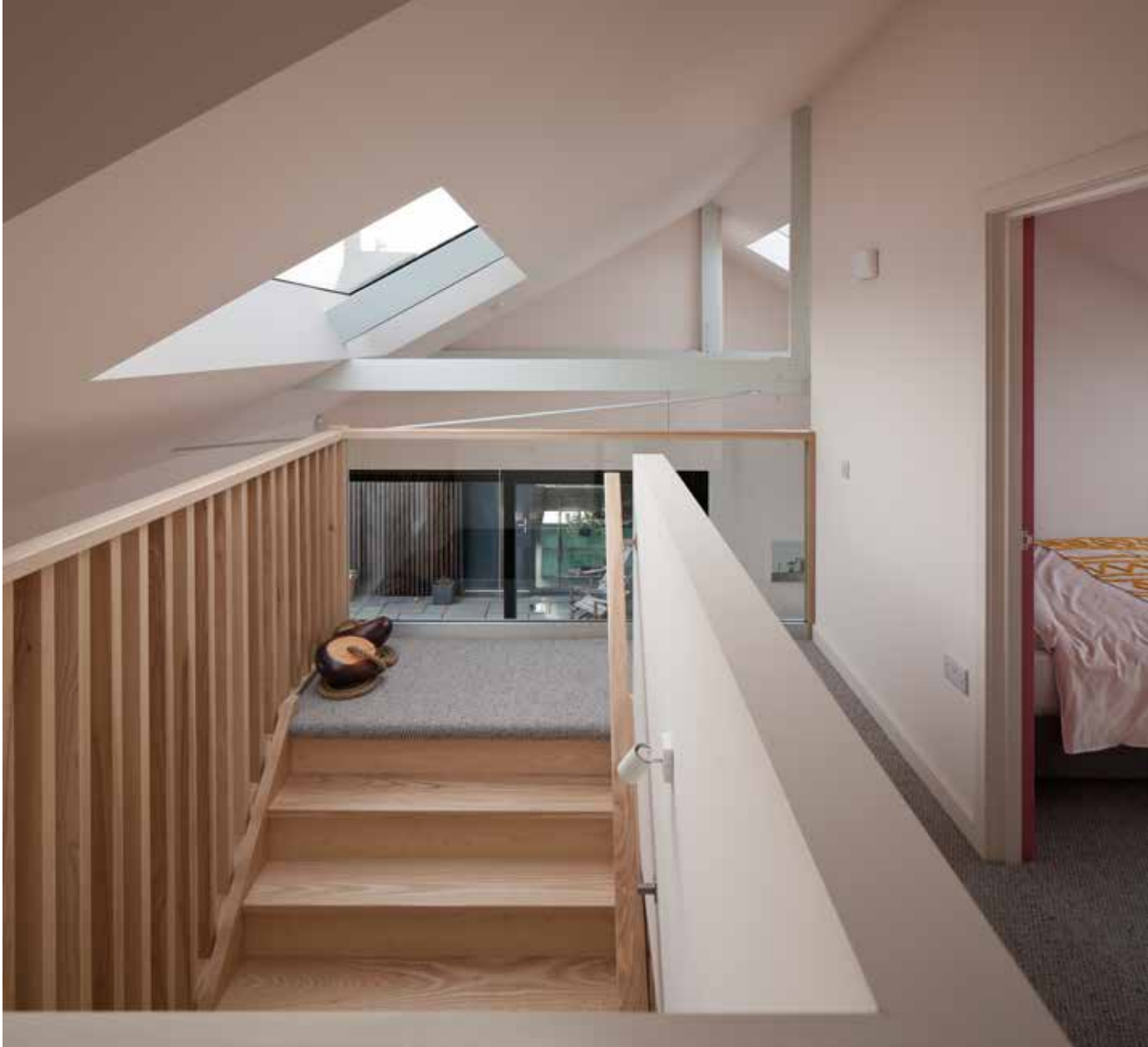
ABOVE AND ABOVE LEFT Designed by Christine, the American ash staircase was made in a workshop by a local fabricator and assembled on site by her joinery team
